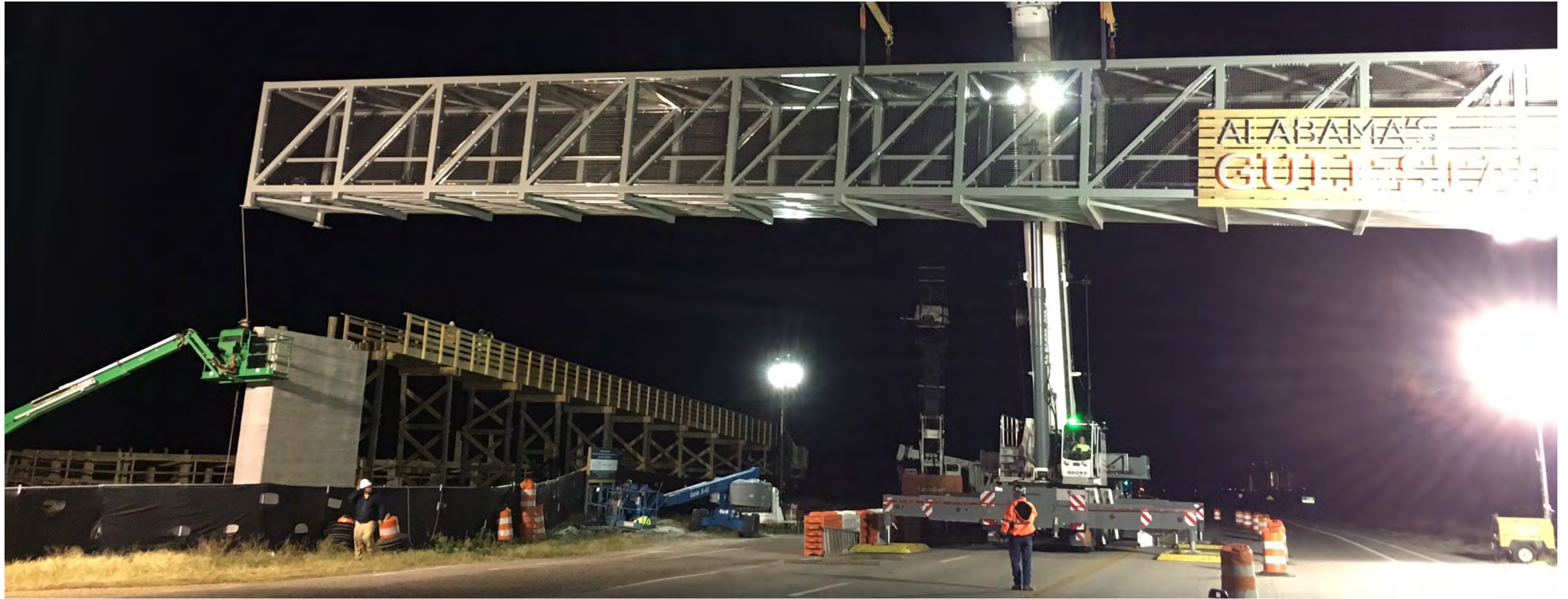
East Pedestrian Bridge Construction
