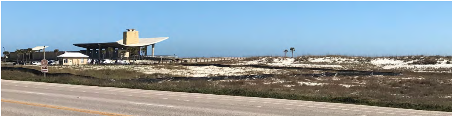
Site Protection in place
