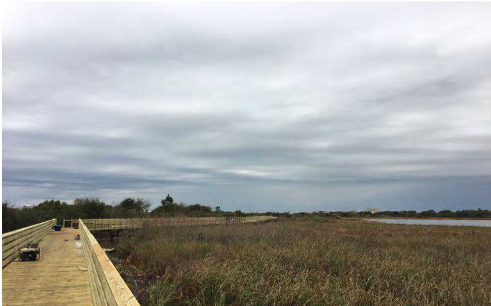
Beach Mouse Bypass Construction
