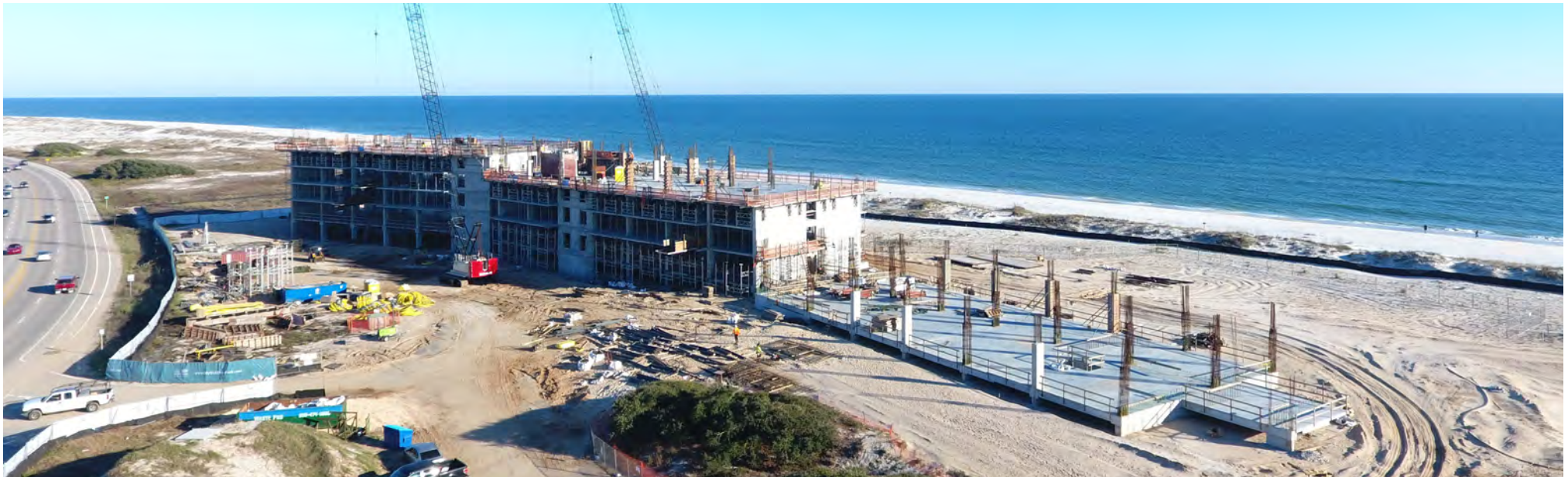
Lodge Construction Progress - Feb 23, 2017
